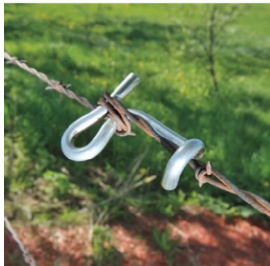
Proper repairs can ensure the integrity of the fence wire. Upper Left -Splicing clip, Upper Right-“Western Union” splice Other repair techniques can create future issues. Bottom Left – twisting clip puts bends in the wire Bottom Right – looped wires create a bend in the wire
